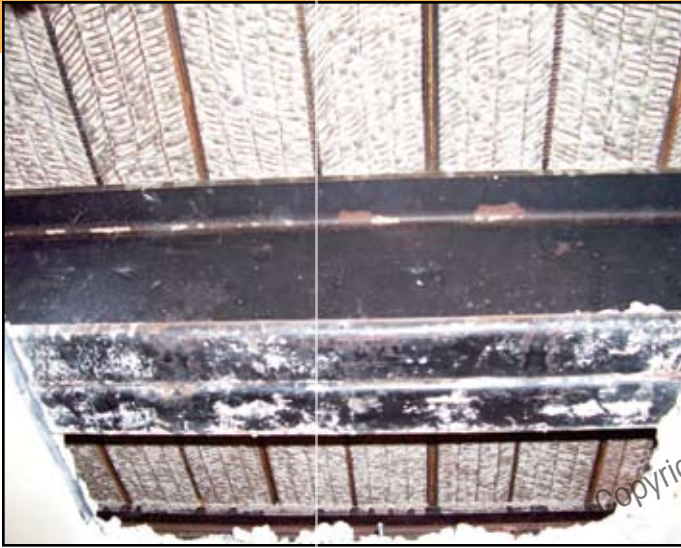
2006 photo of floor joists in Virginia Baptist Hospital during renovation. Metal lath was draped across top flanges of beams and used to support concrete fill.
