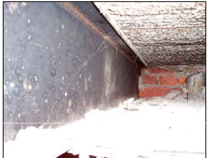
End support of cold-formed steel beam in brick masonry wall, Virginia Baptist Hospital. Construction completed around 1925.
