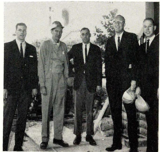
PASADENA PROJECT—At Mutual Savings & Loan building in Crown City: Pete Berger of Berger Bros., plastering contractors; J. J. Devlin, superintendent for Del E. Webb Company; Paul Berger; George L. Throop Jr. of material supply firm; Terry Golnick of United States Gypsum.
